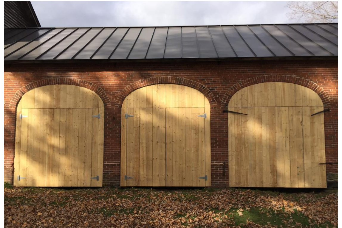
Replicated severely deteriorate doors and hinges
